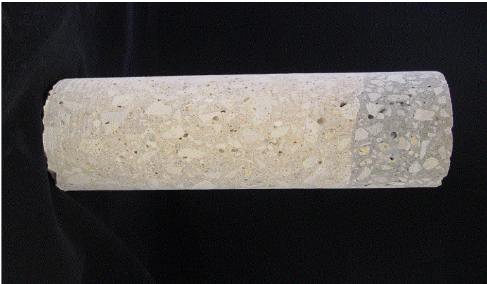
Figure 2. Core 2 taken from the same bridge, also 4" diameter. This core shows no damage. The analysis was done from the surface to the bottom in 1 cm increments.
